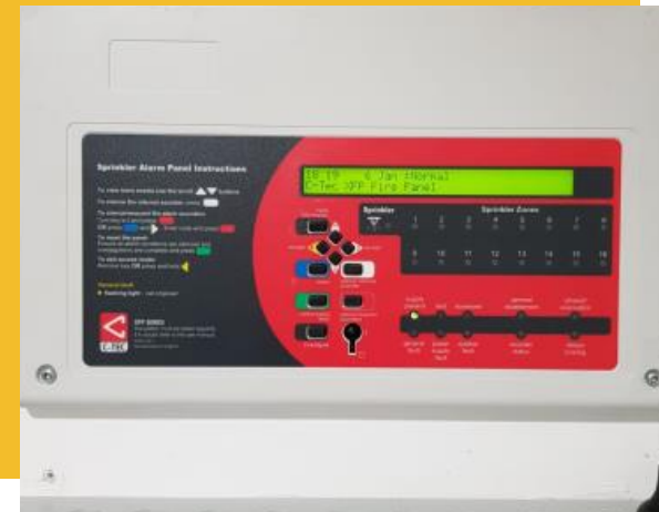
Sprinkler Alarm Panel
